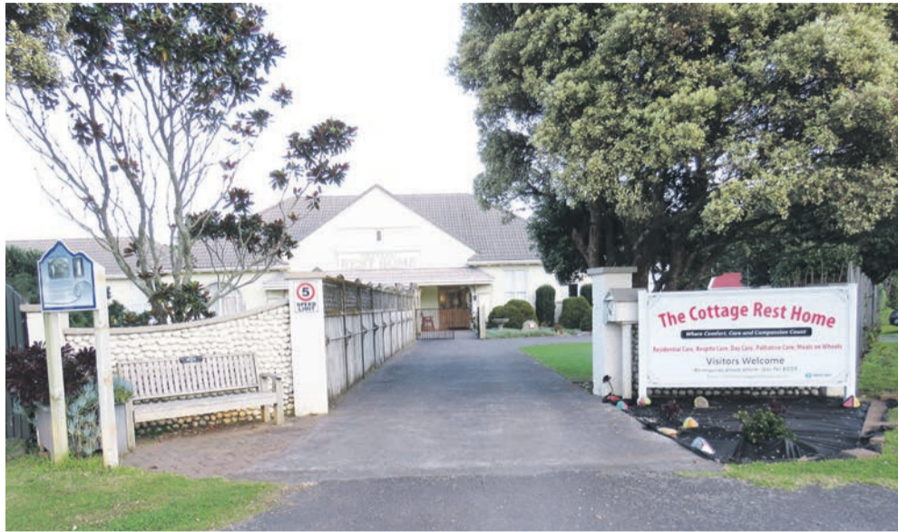
Opunake's Cottage Rest Home.
